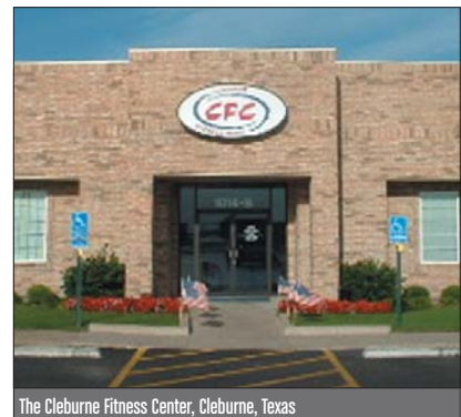
The Cleburne Fitness Center, Cleburne, Texas
